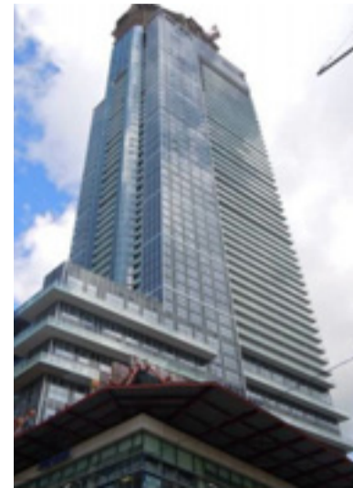
At Yonge and Gerrard Sts., 78-storey Aura is Canada's tallest condo tower.
